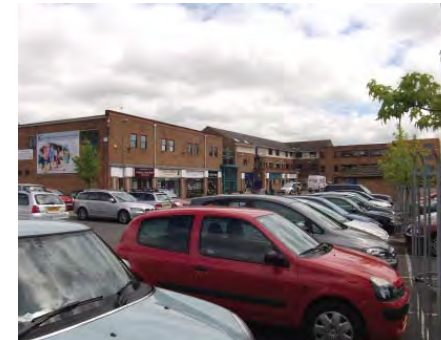
Figure 4.4 Surface car parking
