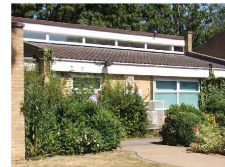
Figure 4.7 Health centre, Exeter Close
